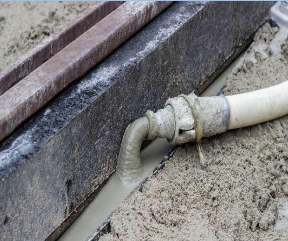
Grouting mortar is used to grout machines and metal structures and/or for structural fills. The additive to use in its formulation is **Pentamix N**.
