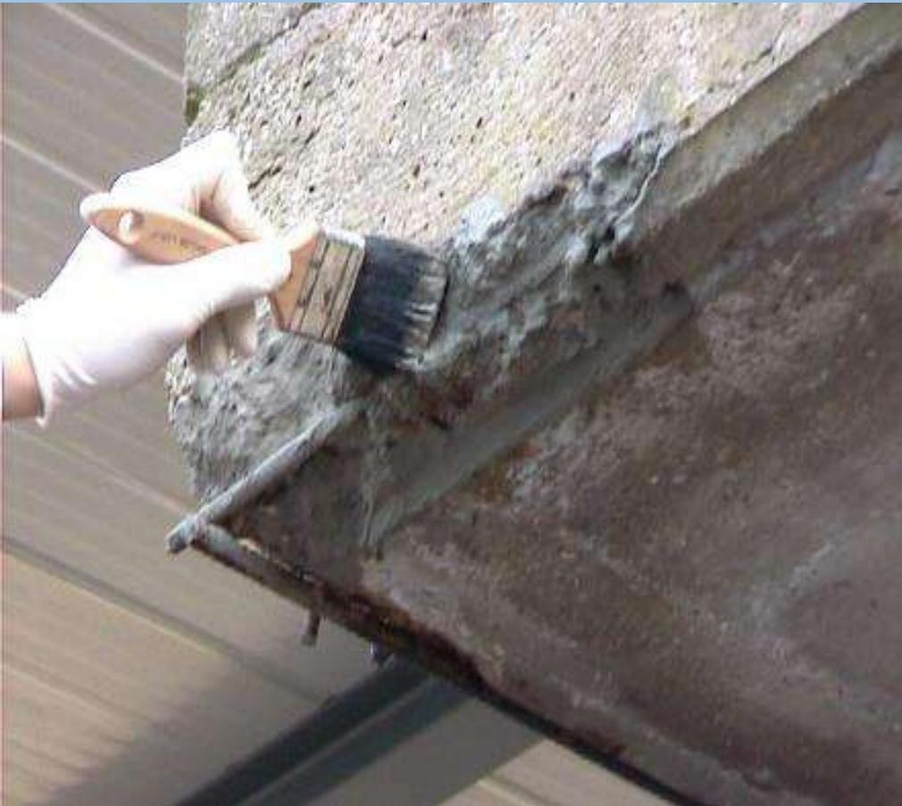
**Antiox L 30:** it is an antioxidant liquid for the protection of the iron rods.
