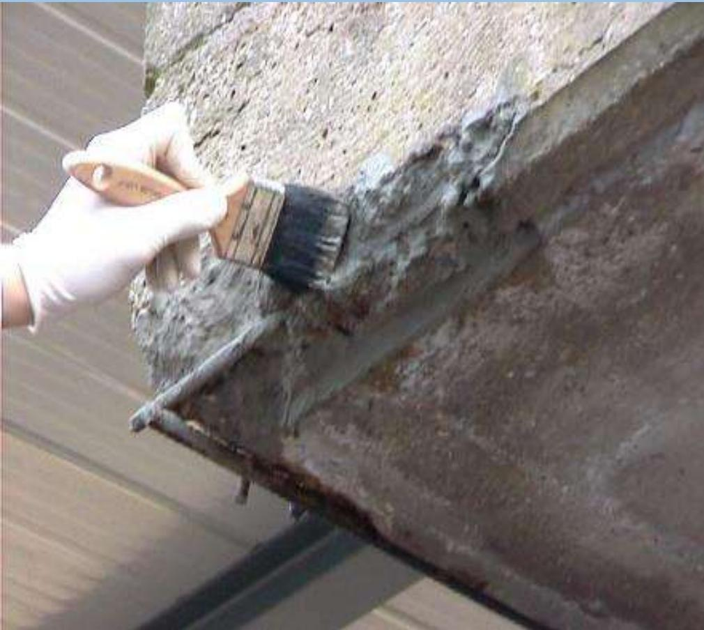
**Pentamix FER 2:** is an additive in powder form that hinders the corrosion of the rods and makes the application of the grout easier and more effective.
